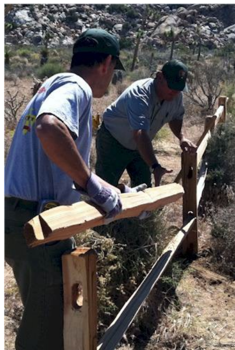
The OA hard at work replacing a split-rail fence in Joshua Tree. (Photo: M. Hare)
